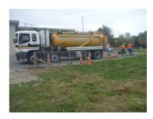
Example of use of hydro excavation by SCL in Timaru Substation – Note – hydrovac both sides of trench, mark large X on ground at service locations so that digger operator has visual alert when approaching buried service.
